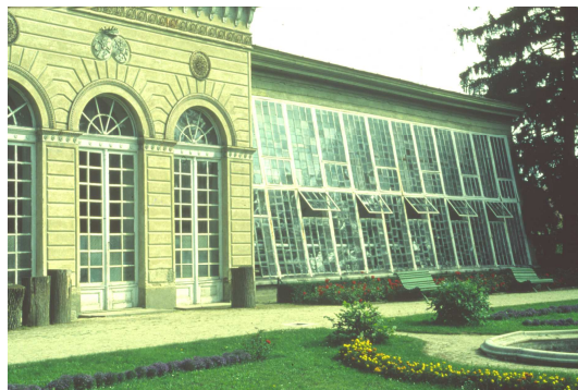
Greenhouse, Palace Garden of Telc, ca. 1800
